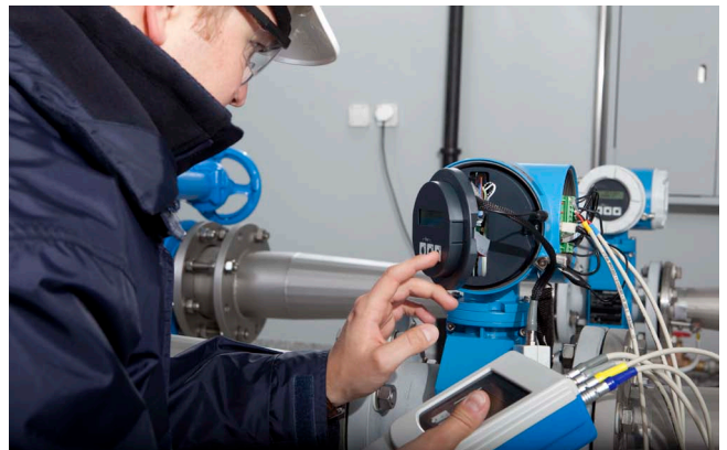
Fieldcheck: traceable verification in installed condition.
