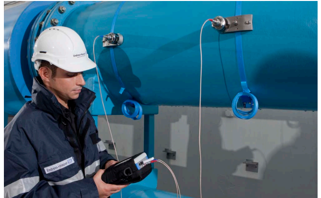
Ultrasonic clamp-on: comparative measurement without interrupting the process
