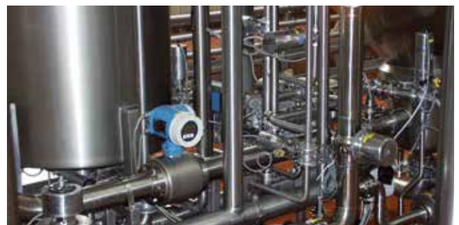
The Rothaus Brewery well equipped by Endress+Hauser instruments
