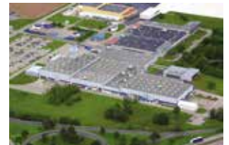
Product Center Wetzlar Germany Data Acquisition, Temperature, R&D, Production and Calibration
