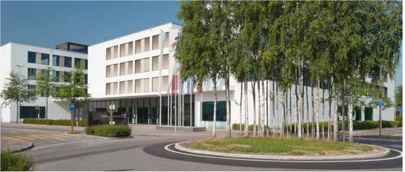
Endress+Hauser Headquarters in Reinach, Switzerland
