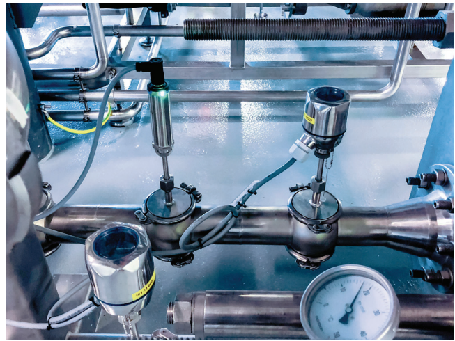
Installed iTHERM TrustSens sensor at the brewery
